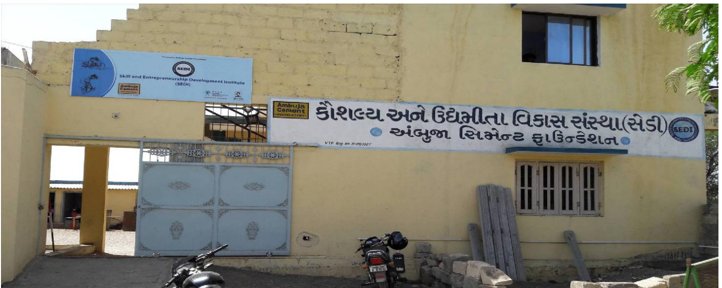
Figure 10: Skill & Entrepreneurship Development Institute (SEDI), Ambuja Cement Foundation, Kodinar
