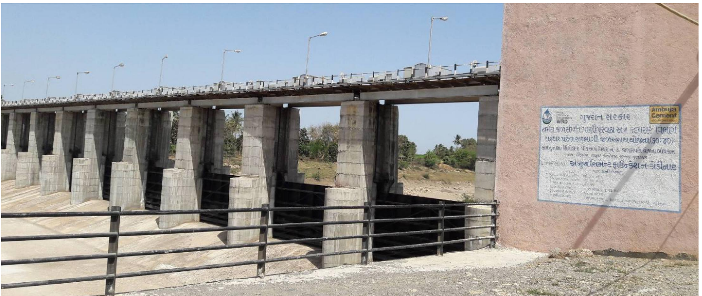
Figure 9: Check dam constructed at Kodinar by Gujarat Government & Ambuja Cement Foundation
