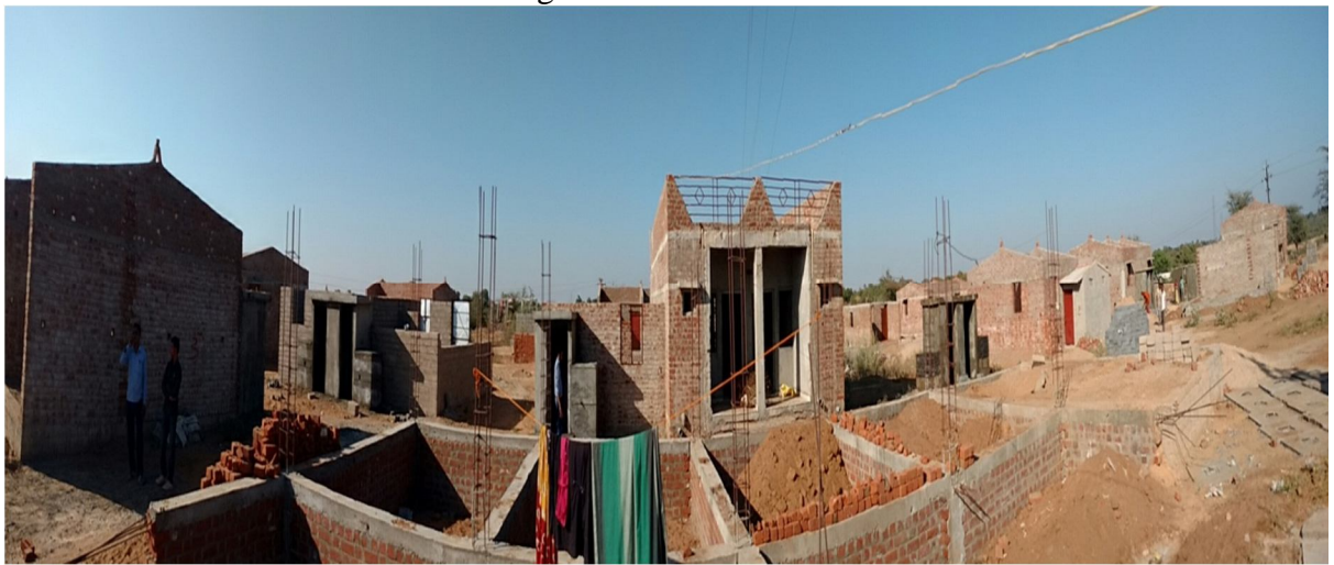
Fig 4. Ongoing Project Site
