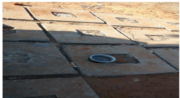
Fig 2. Casting of Water Tank Plates
