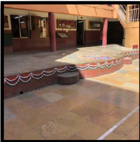
Stage area has irregular steps of over 150mm. Front edge of stage needs non-slip contrast.
