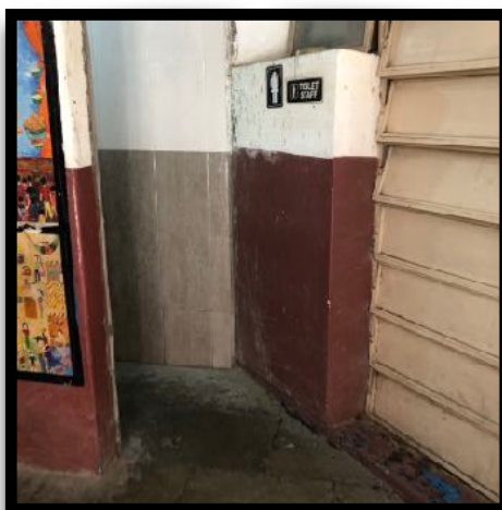
Toilet blocks are reached via a single step level change and narrow entrance.
