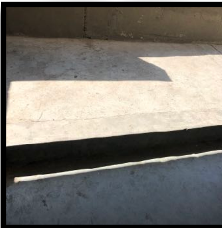
Single step onto glossy surface on 1st floor corridor to toilets. Non-compliant.
